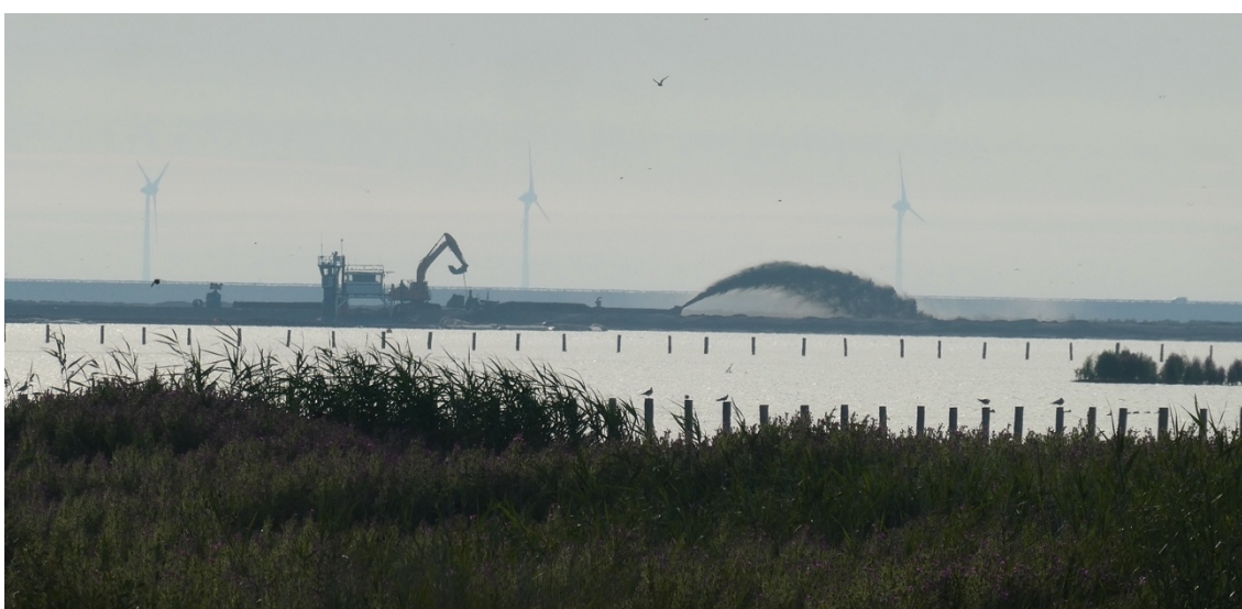
New basins filled with local silt from the freshwater lake were still constructed in 2021-2022.
